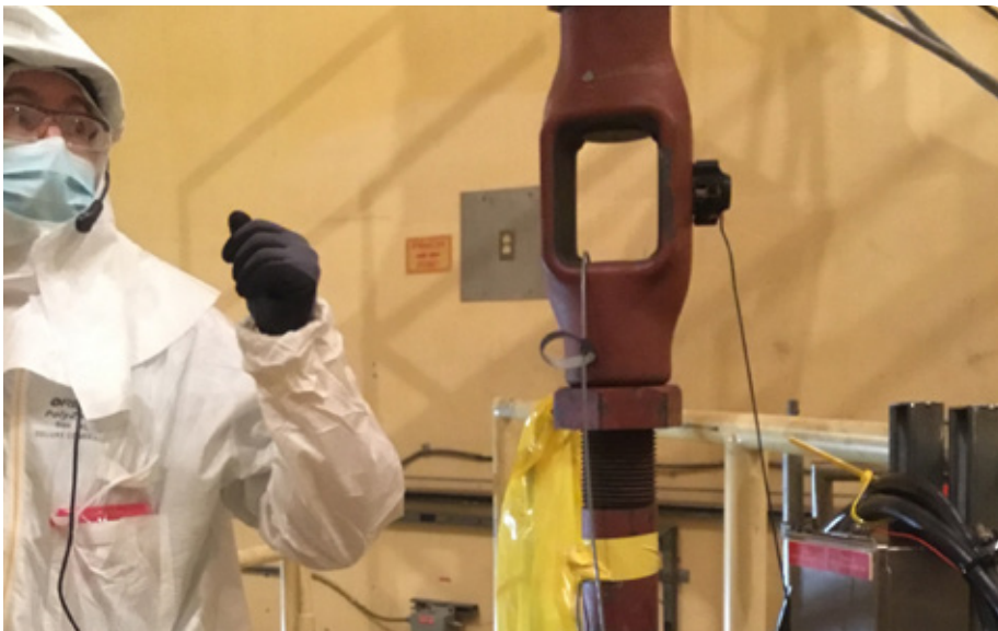
FIGURE 2. Lift rig turnbuckle outfitted with AE sensor.
