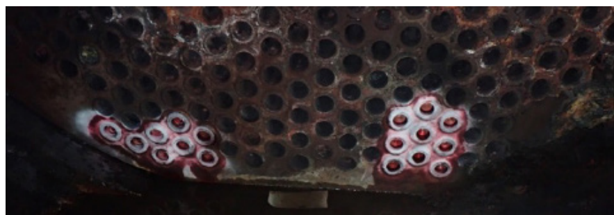
(a) Plugged tube-to-tube joints
