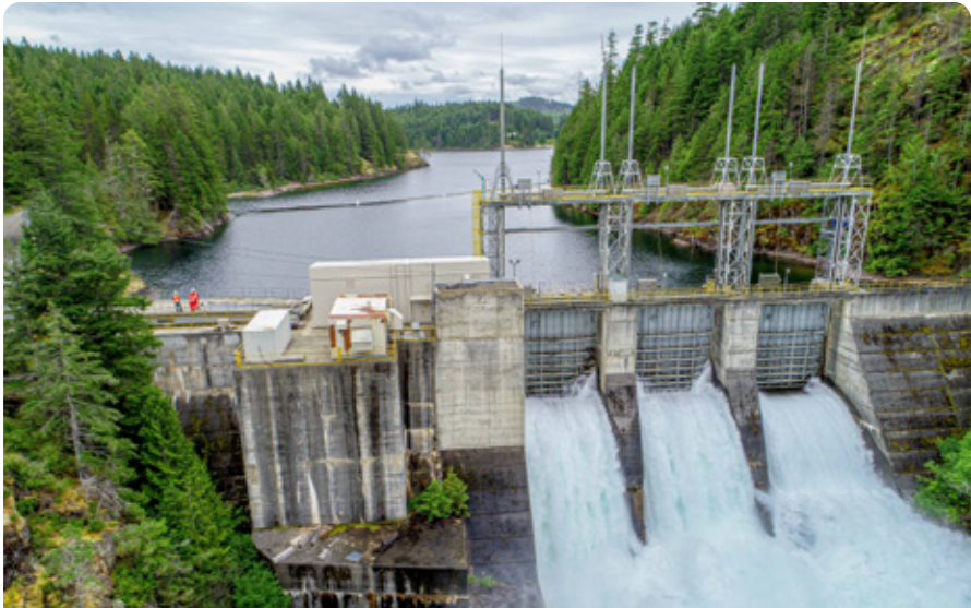
FIGURE 1. Ladore Dam Spillway, Image courtesy BC Hydro Ref: https://www.mycampbellrivernow.com/wp-content/uploads/2021/01/John-Hart-Dam.jpg
