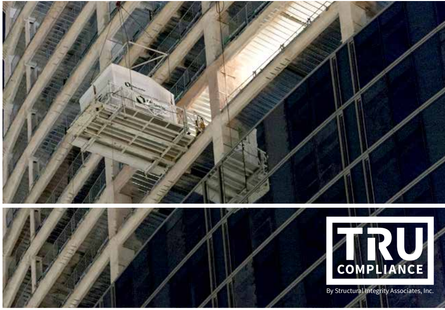
FIGURE 3. Modular bathroom being installed at Wilshire Grand Hotel, Los Angeles 2
